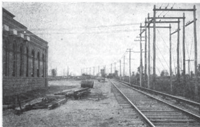
FIG. 11.—LINE ANCHORAGE AT POWER STATION, SCIOTO VALLEY.
